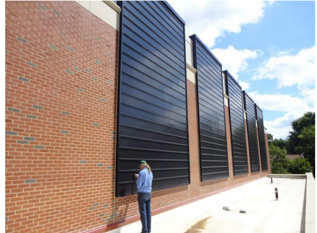
Image 8: Solar Wall – courtesy of http://www.taitem.com/news/lou-cherry-road-solar-wall-1/
