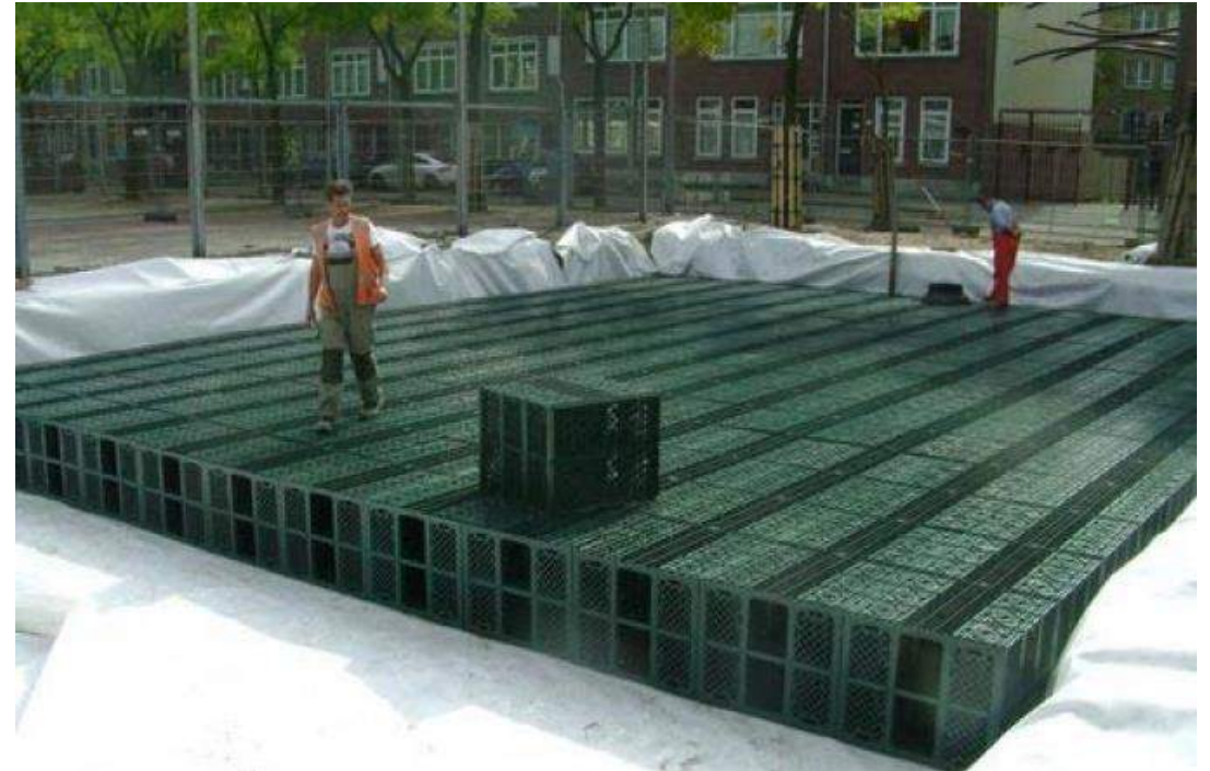
Image 12: Installation of water storage structure below playing field
